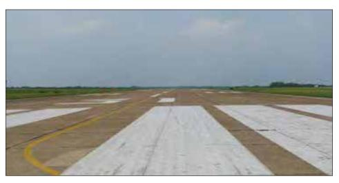
displacing the Runway 31 landing threshold by 500 feet. In order to maximize take-off length for Runway 13, the departure RPZ could begin no closer than 170 feet northwest of the current runway end.
